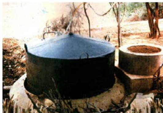
Fig: Indian floating drum gas holder
